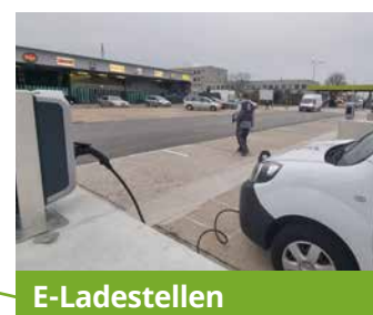
Hypercharger Schnellladestation
